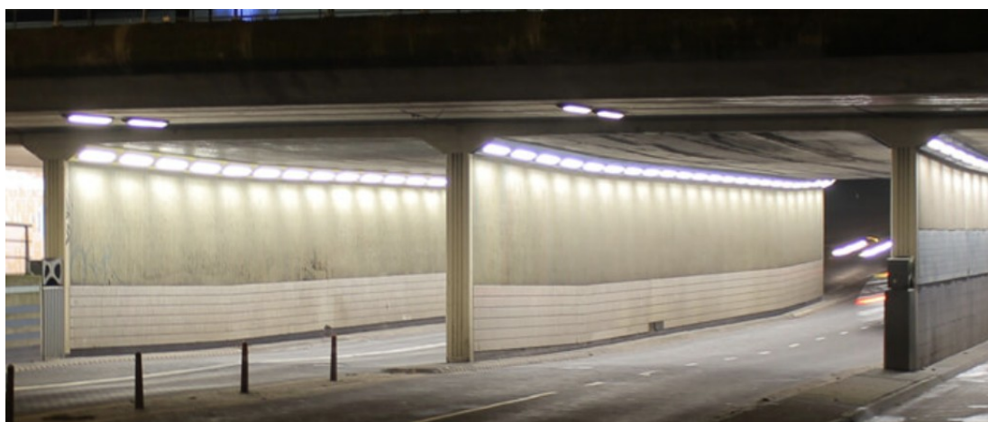
LED verlichting in tunnel
